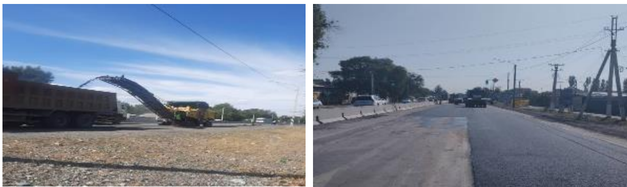
Figure 3 Milling and laying wearing course, removing rutting
