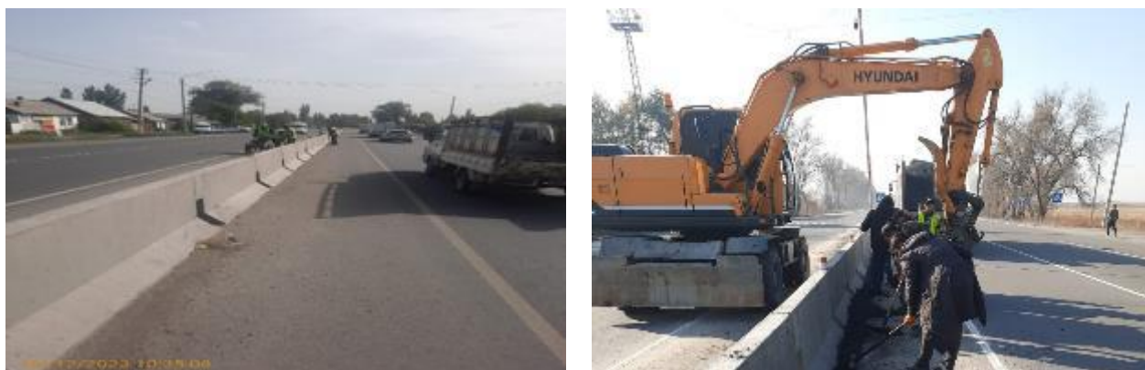
Figure 9 Cleaning and removal soil waste near parapets
