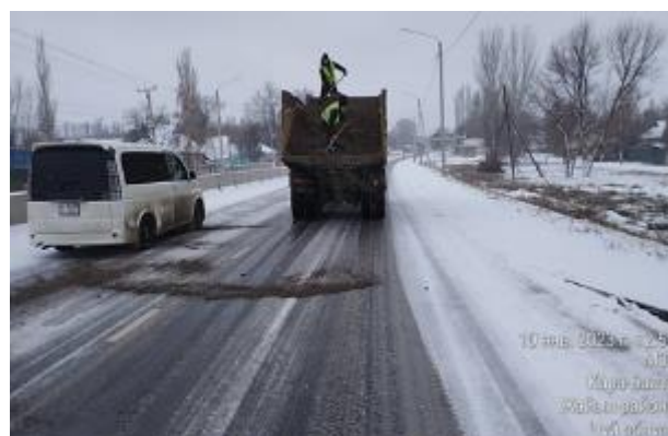
Figure 8 Sand sprinkling on the road. Control of ice
