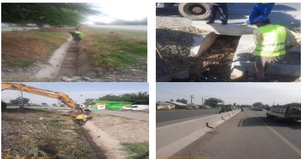
Figure 4 Cleaning of culverts and parapets from accumulated soil
