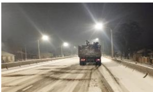
Figure 8 Sand sprinkling on the road. Control of ice
